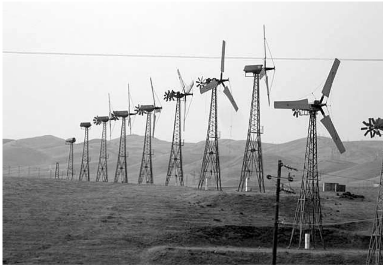
Smaller wind turbine blades turn just at cruising height for the raptors of Altamont Pass, a flat, sloping terrain with strong steady winds located east of San Francisco Bay. The open lattice towers also invite nesting. An estimated 1,700 to 4,700 birds are killed every year, or around one bird for every one or two windmills per year. Wind proponents say taller towers will help solve the problem, but others say the jury is still out. Photo by Bill Kovarik
